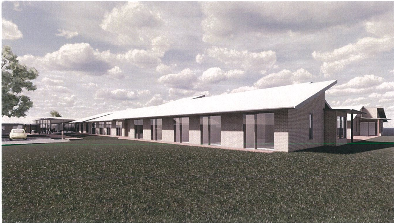
2 View of New Wing from North-East 1:1
